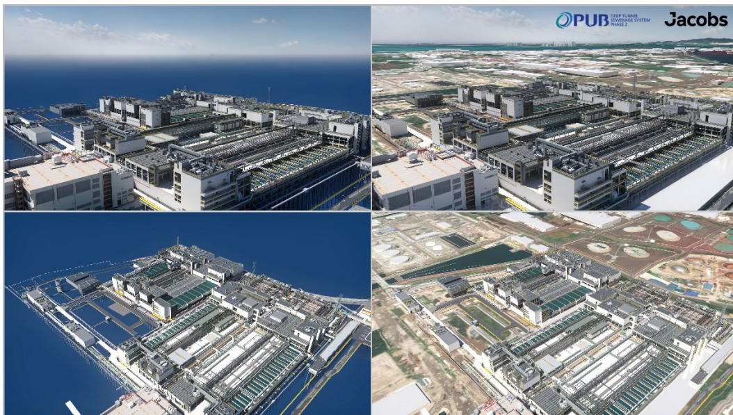
Tuas Water Reclamation Project. Image courtesy of PUB, Singapore's National Water Agency, and Jacobs.
